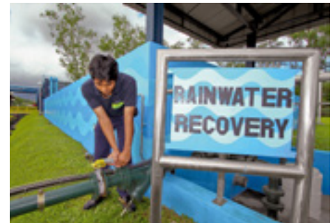
An example of environmental awareness at our Lipa factory in the Philippines, which has a system to collect rainwater from catchment areas and then reuse it in areas such as the cooling tower.
